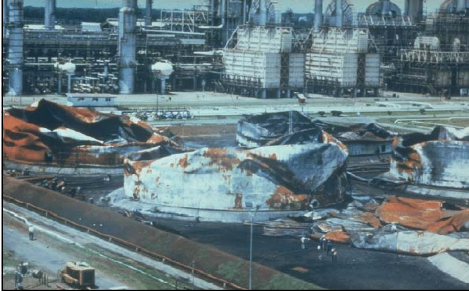
Oil refinery Pertamina, Cilacap/Java, 1995: 7 tanks burned out due to a lightning strike
